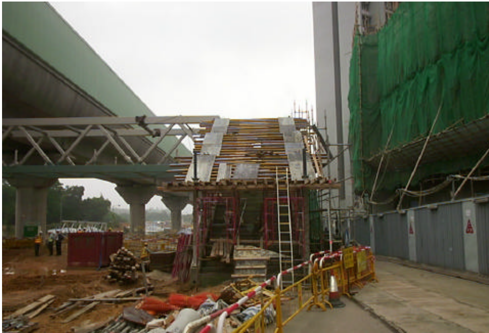
Date: 1 April 2004 Works: Construction of Footbridge Location: Near Lee Wing House
