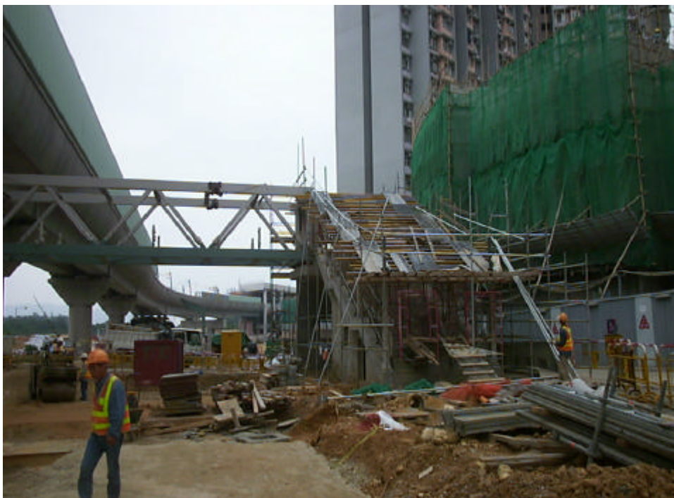
Date: 8 April 2004 Works: Construction of Footbridge Location: Near Lee Wing House
