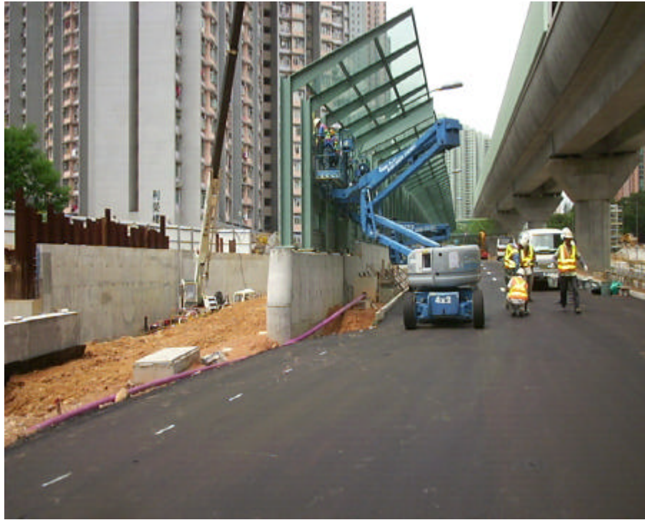
Date: 8 July 04 Works: Noise Barrier Work Location: Near Lee Wing House
