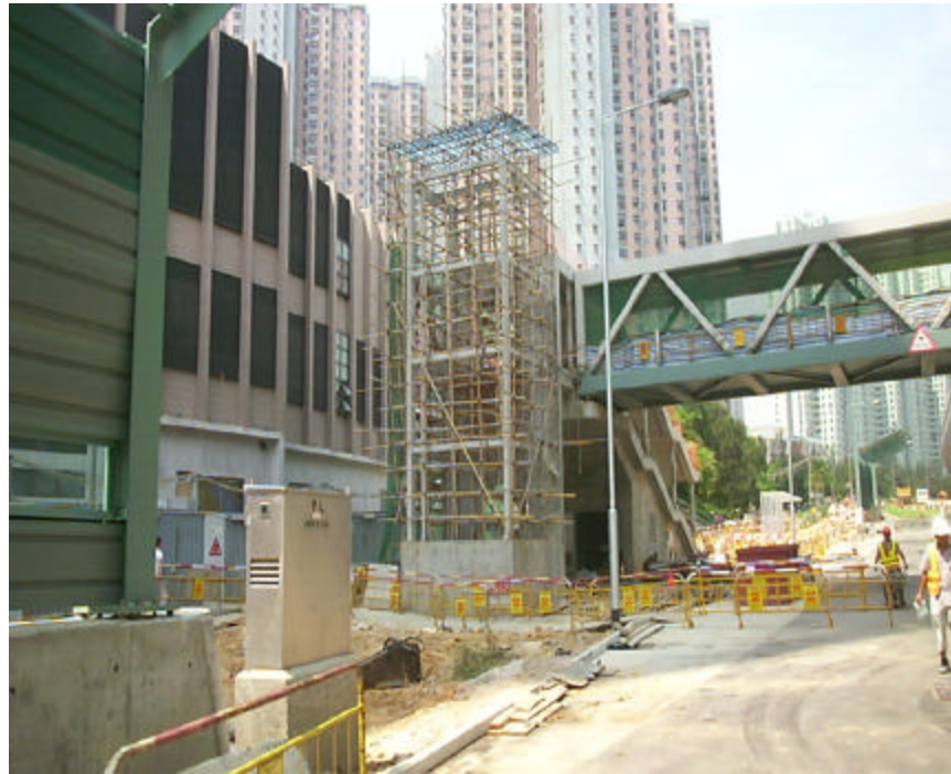
Date: 2 July 2004 Works: Footbridge Construction Location: Near Lee Wing House
