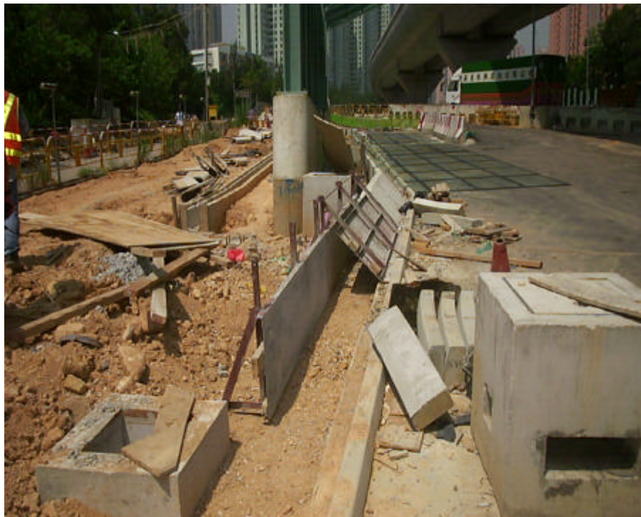
Date: 2 July 2004 Works: Road Work Location: Near Kam Lung Court
