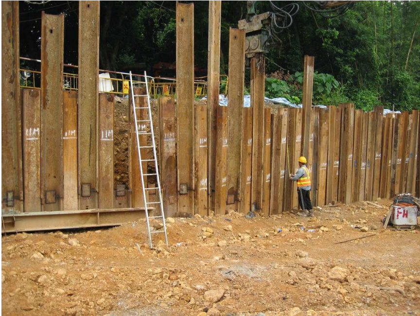
Date: 26 August 04 Location: Near Subway 2 Works: Sheet Pipe Work
