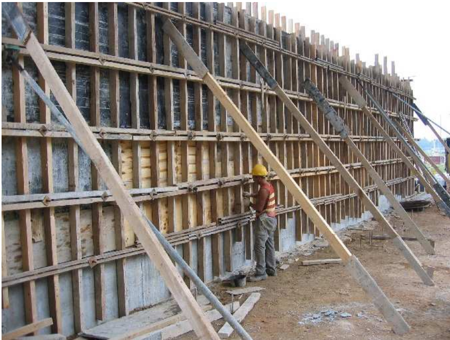
Date: 26 August 04 Location: Near Lee Wing House Works: Retaining Wall Work
