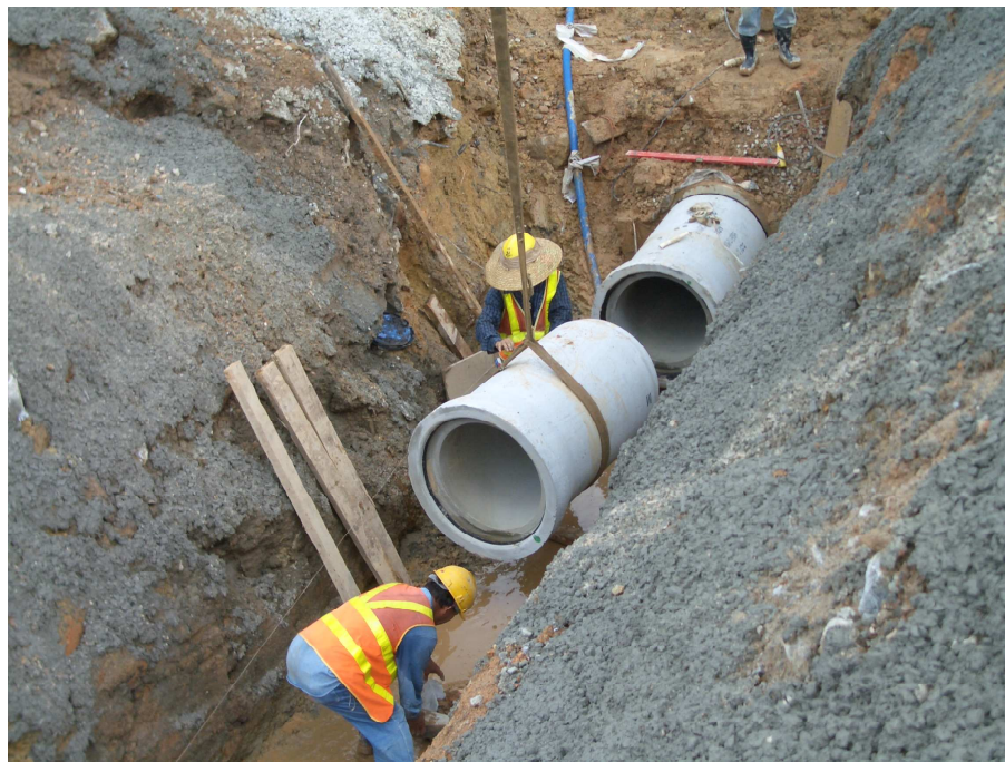
Date: 26 September 2004 Location: Proposed Residential Development at DD206
