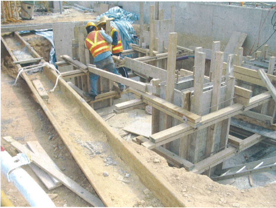
Date: 27 January 05 Works: Drainage works Location: Proposed Residential Development at DD206
