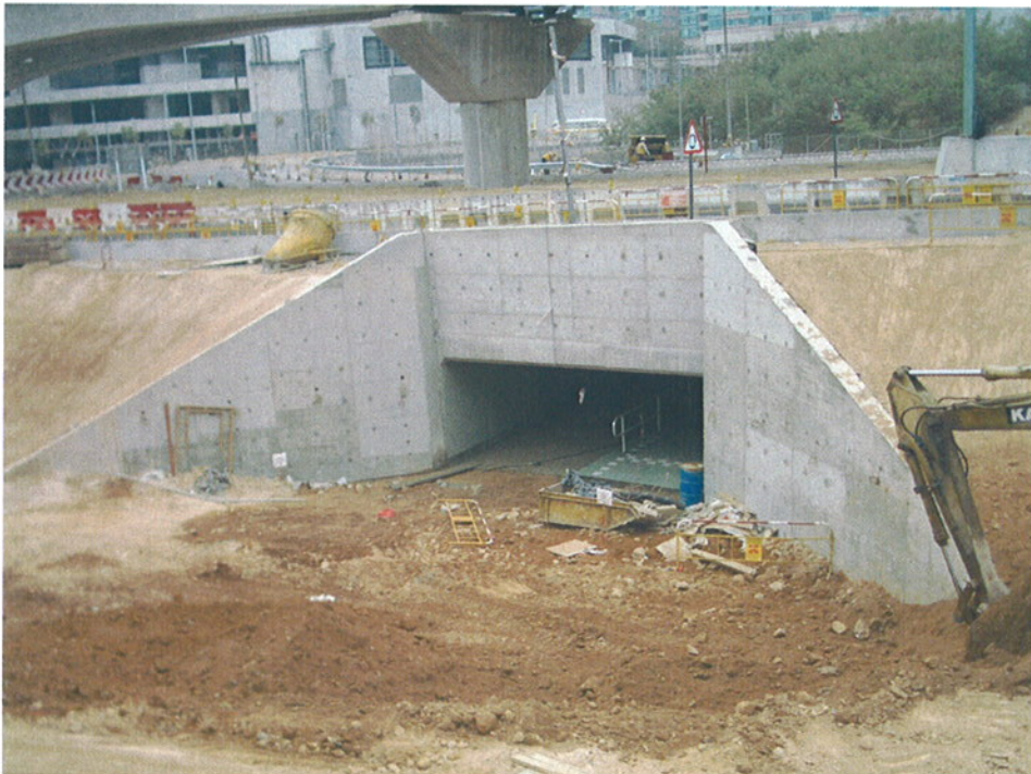
Date: 20 January 05 Works: Tunnel Work Location: Proposed Residential Development at DD206
