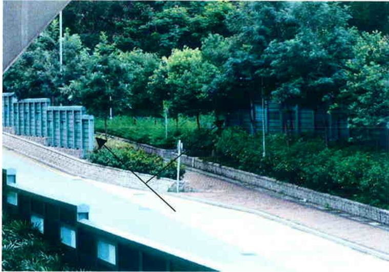
The gap between the edge of noise barrier and the lift
