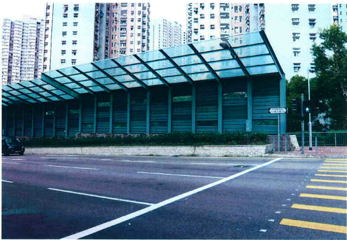
Noise Barrier Type IV in the Westbound Carriageway of Sai Sha Road near Kam Ying Road
