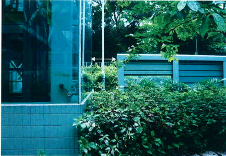
The gap between the edge of noise barrier and the lift
