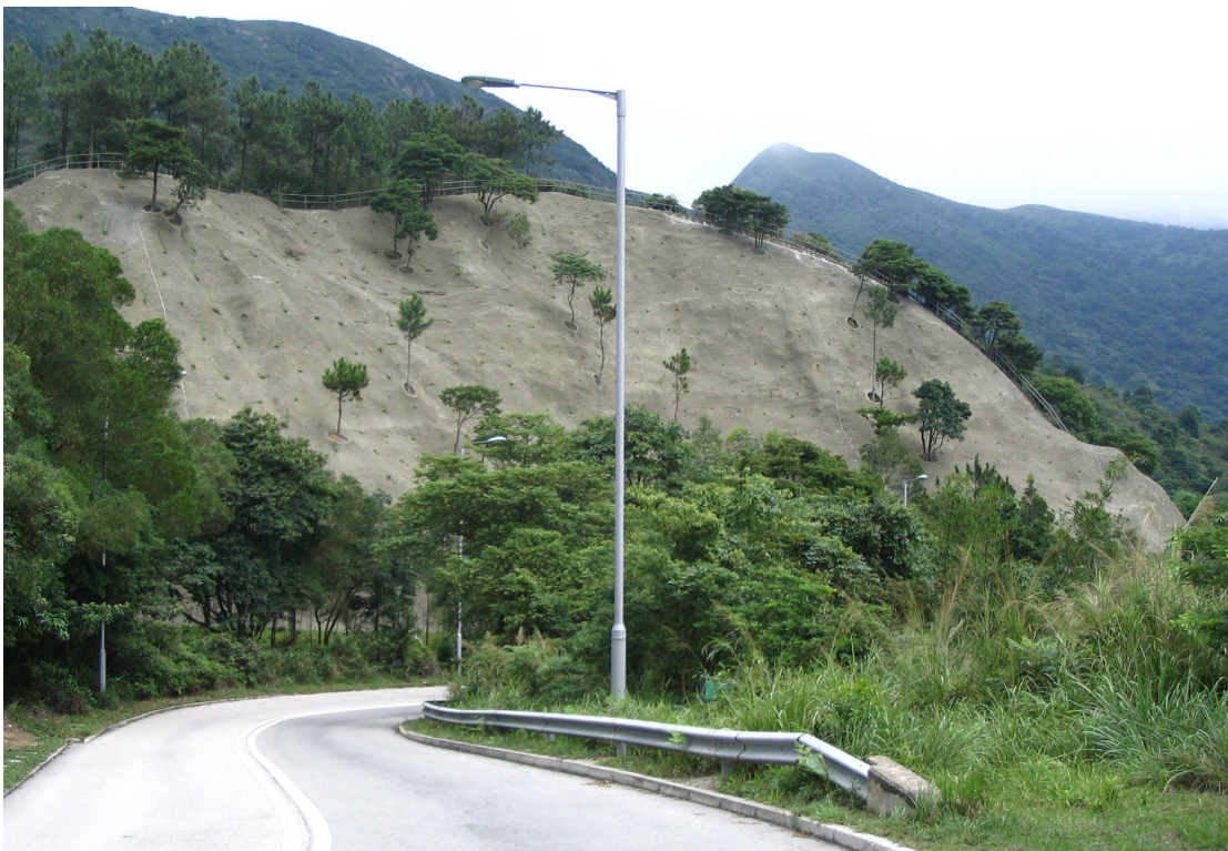
Plate No. 2 General view of the feature from Keung Shan Road
