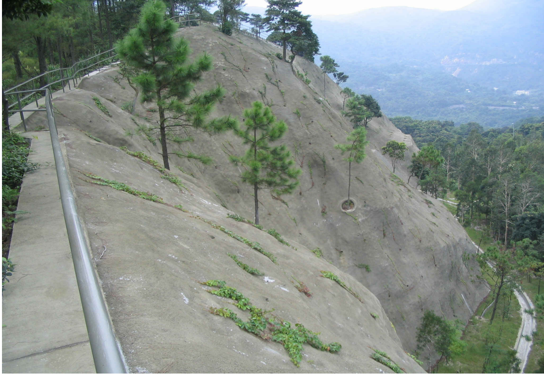
Plate No. 5 Crest view of the slope, with climbers planted over the entire slope surface
