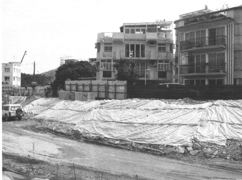
Photo 1: Covering of earth materials with tarpaulin sheeting.
