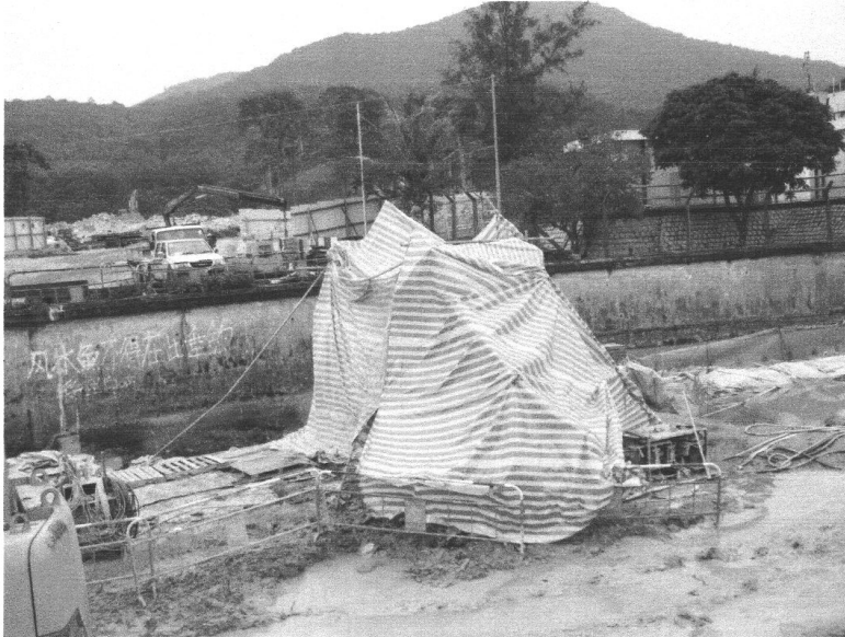
Photo 1: Enclosure of grout mixing plant with tarpaulin sheeting.
