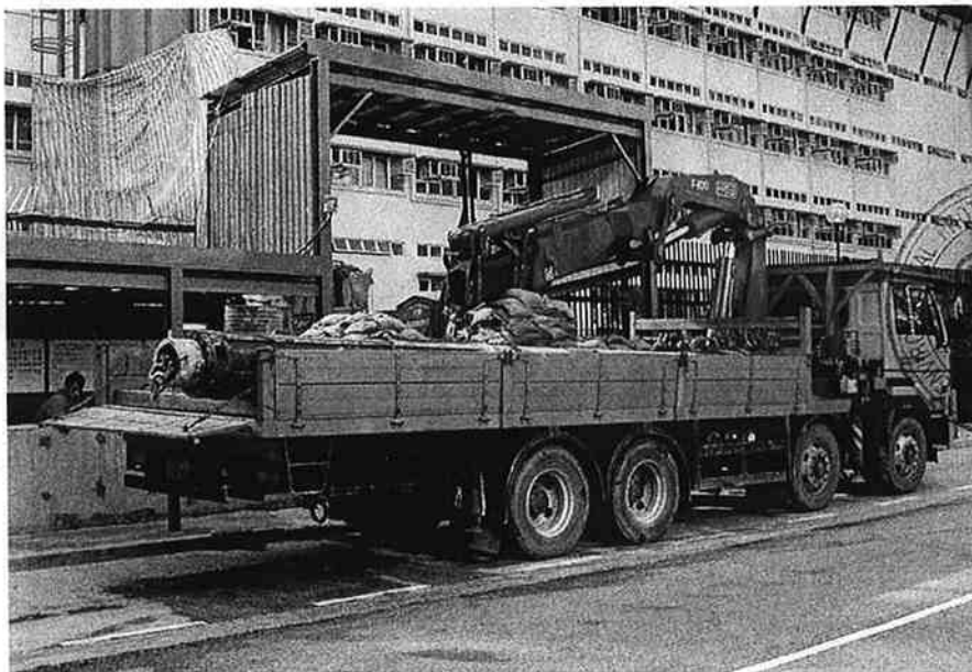
吊臂貨車，總重量 \leq 38 噸 Lorry, with crane, gross vehicle weight \leq 38 tonnes
