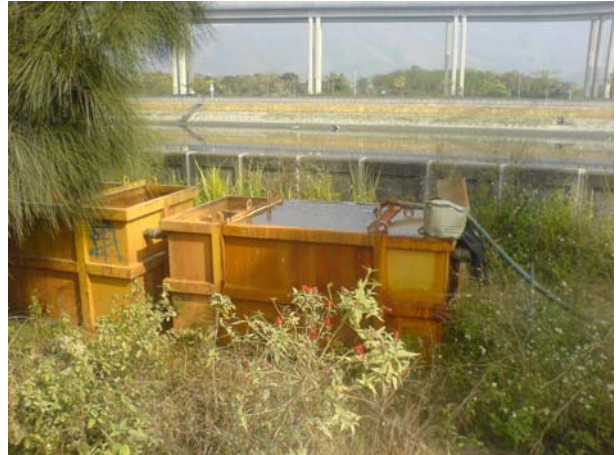
The Contractor was reminded to remove the sediment in the desilting facilities regularly.
