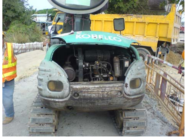
Flap of the excavator should be closed.
