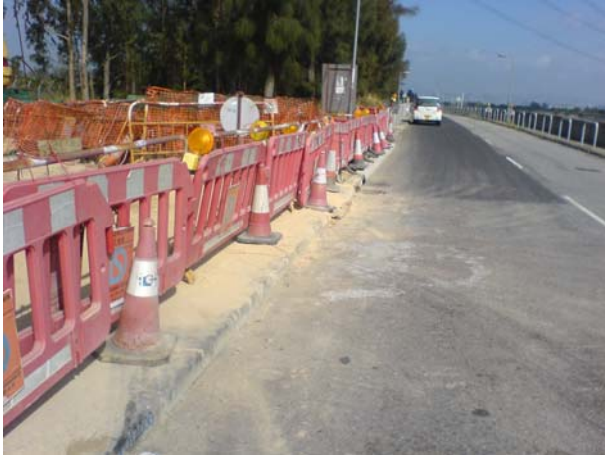
The road should be keep clean.
