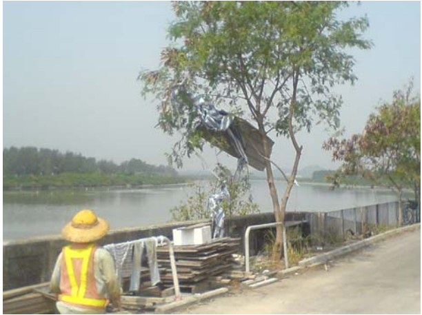
Materials on the tree should be removed to avoid damage to the tree.
