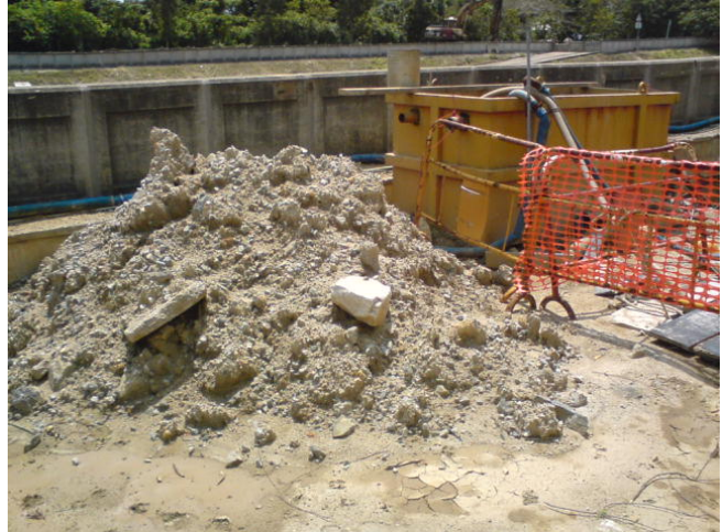
The soil stockpile in the site should be removed or covered with tarpaulin in order to minimize the dust nuisance.
