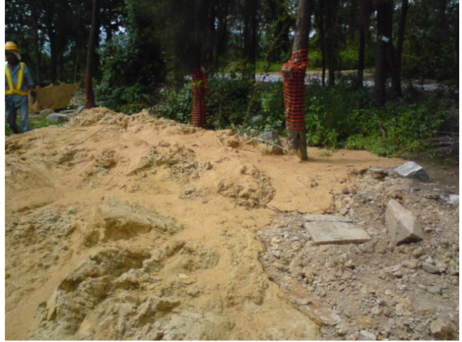
2. Sufficient area should be provided for the preserved trees when the soil stockpile in the site in order to protect against the trees.
