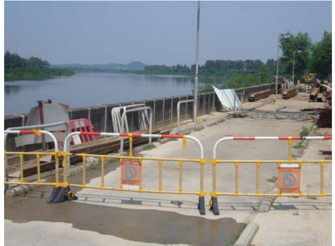
2. Muddy water at Nam San Wai Pumping station was cleared.
