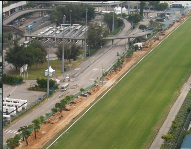
Photo 2: Construction works along the race course.
