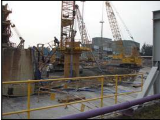
E. 1 Pre-drilling and bored piling at the North Coal Stockyard
