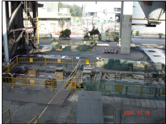
E. 3 Civil foundation for natural gas pipes and fuel oil pipes
