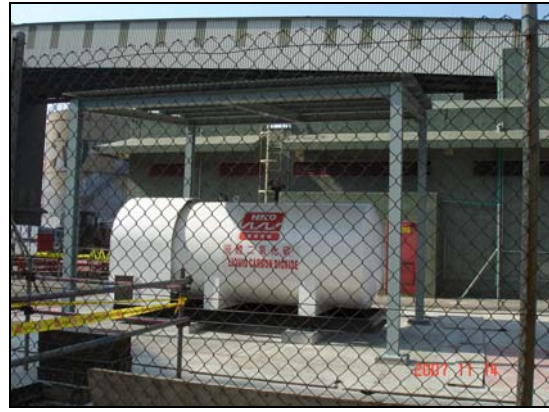
E. 4 Installation of new CO 2 Tank
