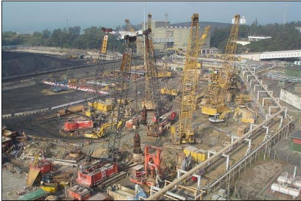
E.1 Pre-drilling and bored piling at North Coal Stockyard
