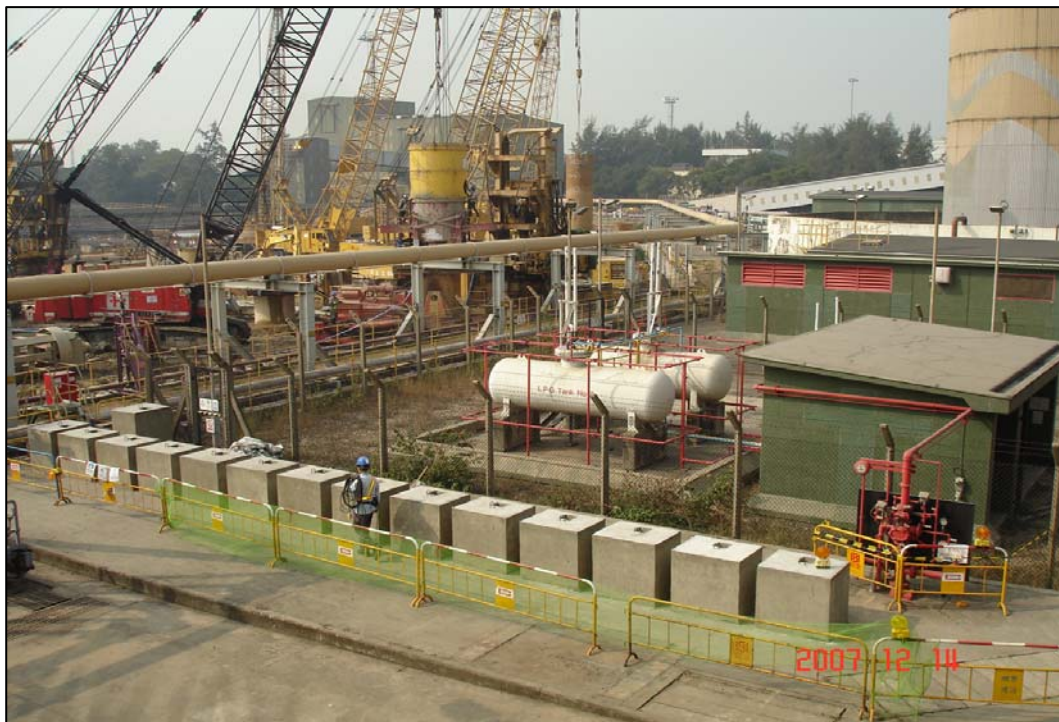
E. 4 Preparation works for LPG compound demolition
