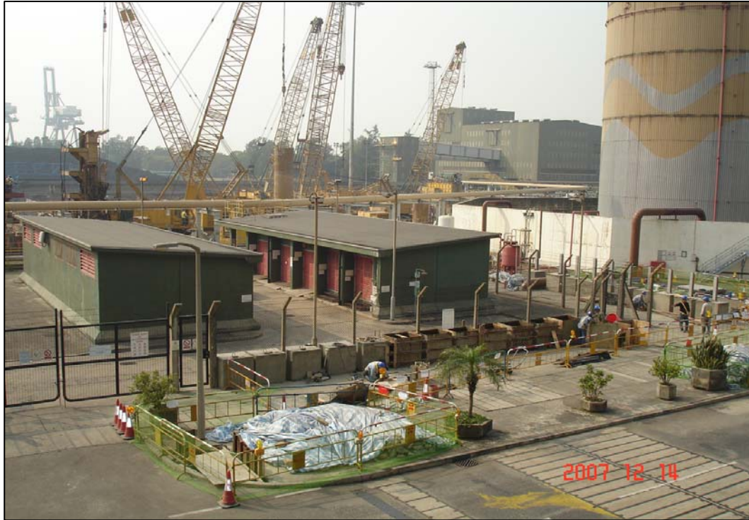
E. 3 Preparation works for DG Stores demolition
