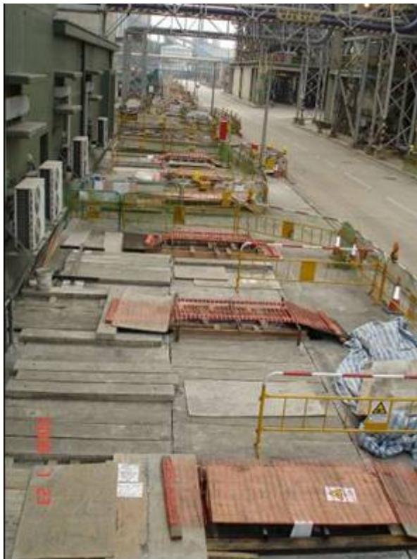
E.4 Construction of pipe support footing for relocation of underground pipe works
