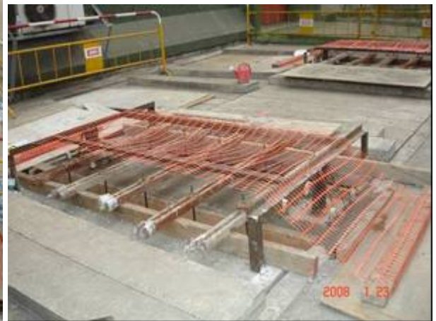
E.4 Construction of pipe support footing for relocation of underground pipe works
