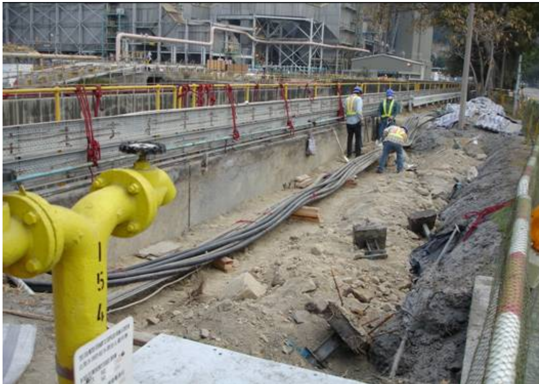
E. 2 Utilities (pipes / cable) diversion
