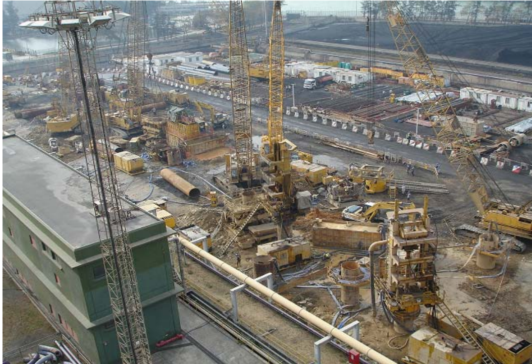
E. 1 Bored piling and pre-drilling at North Coal Stockyard
