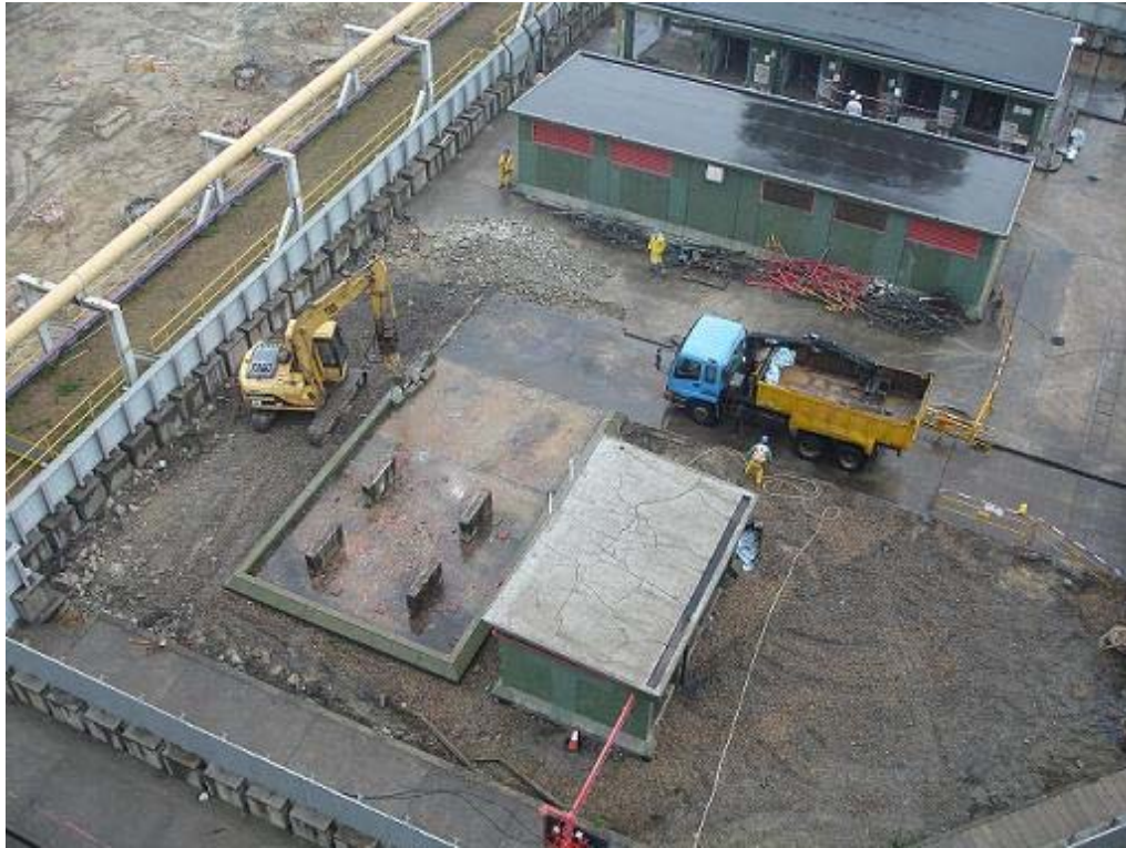
E.3 Decommissioning and demolition of DG Store and LPG compound
