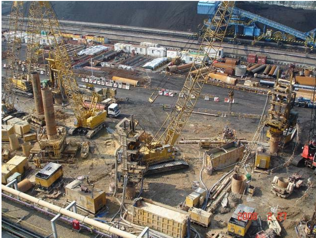
E. 1 Bored piling and pre-drilling at the North Coal Stockyard
