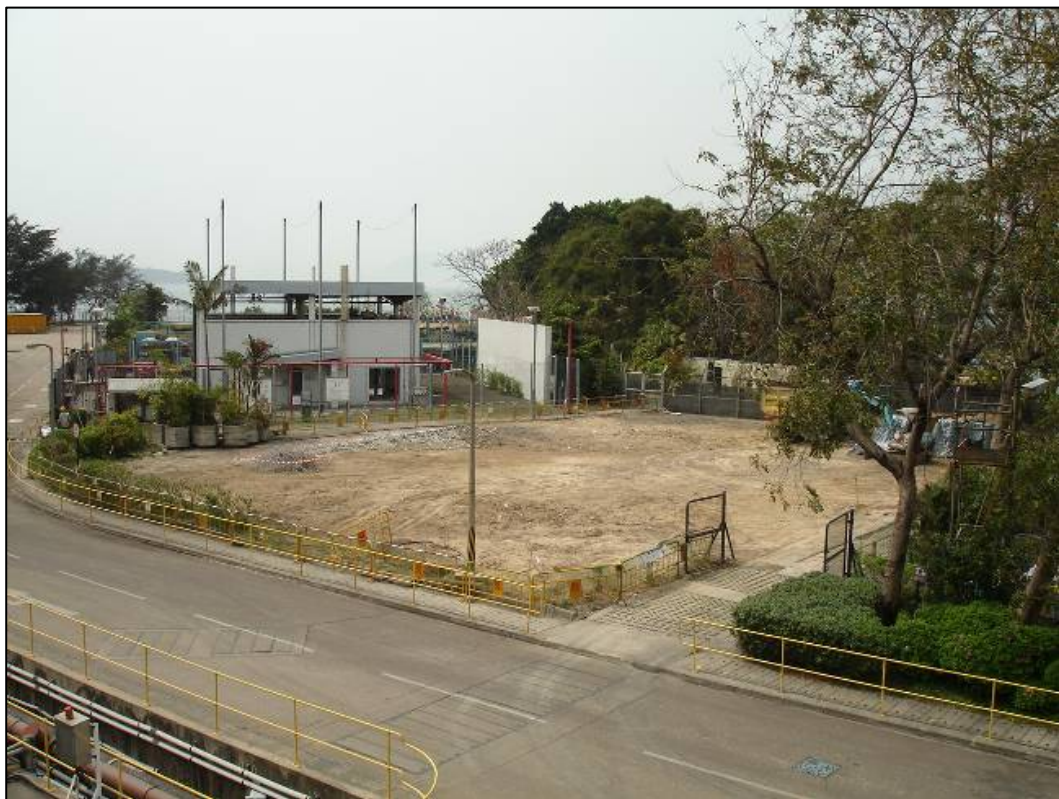
E.4 Site clearance for relocation of Intermediate Pressure Reducing Station
