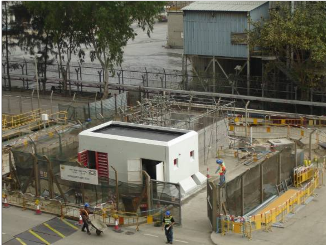
E. 3 LPG Compound relocation and system tie-in works
