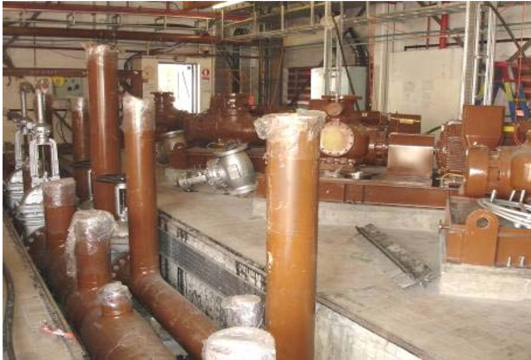
E. 3 Fuel oil system relocation and system tie-in works
