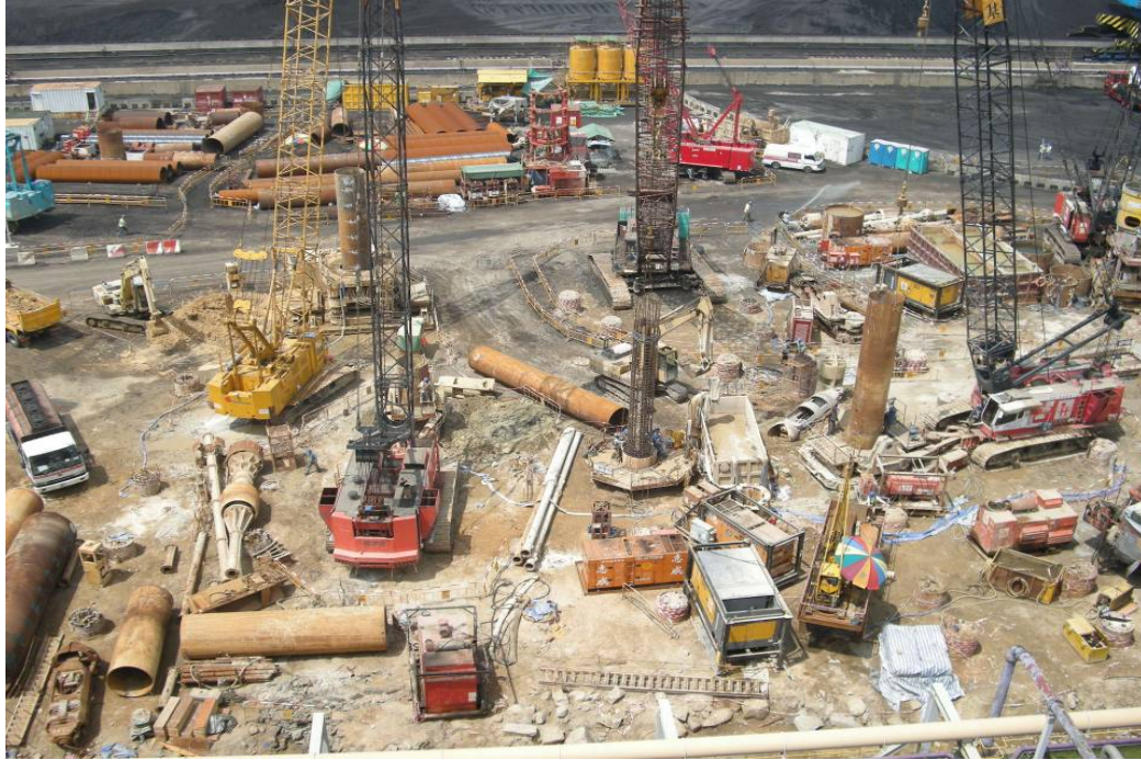
E. 1 Bored-piling and H-piling at the North Coal Stockyard
