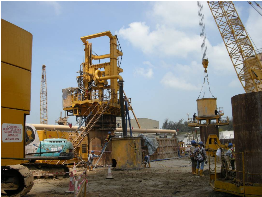
E. 2 Bored-piling at the former D.G. Store area
