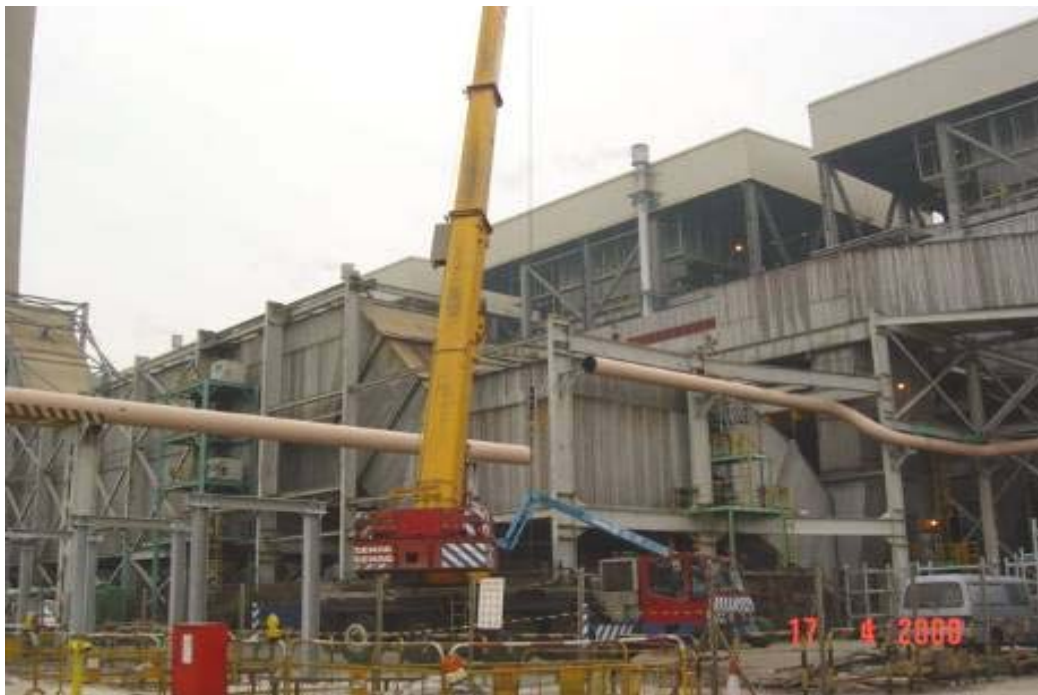
E.4 Demolition of existing natural gas pipeline
