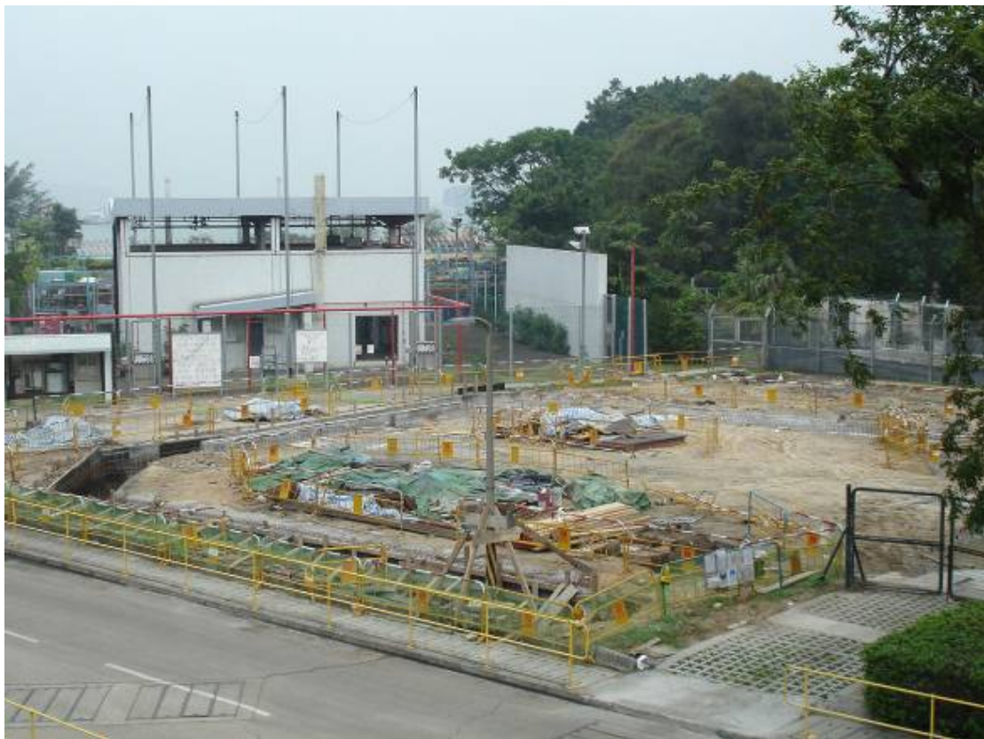
E.4 Foundation works for relocation of Intermediate Pressure Reducing Station
