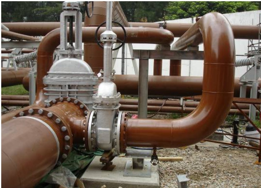
E. 2 Fuel oil system relocation and system tie-in works
