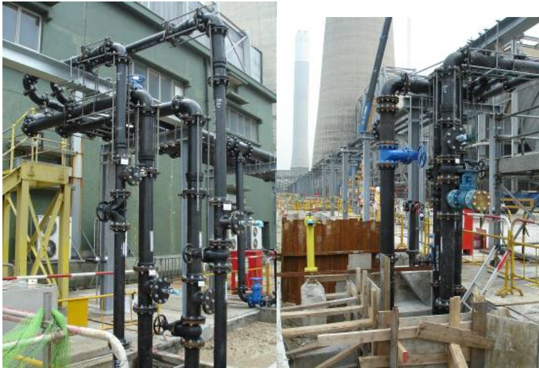
E.3 Relocation of underground utilities pipeline
