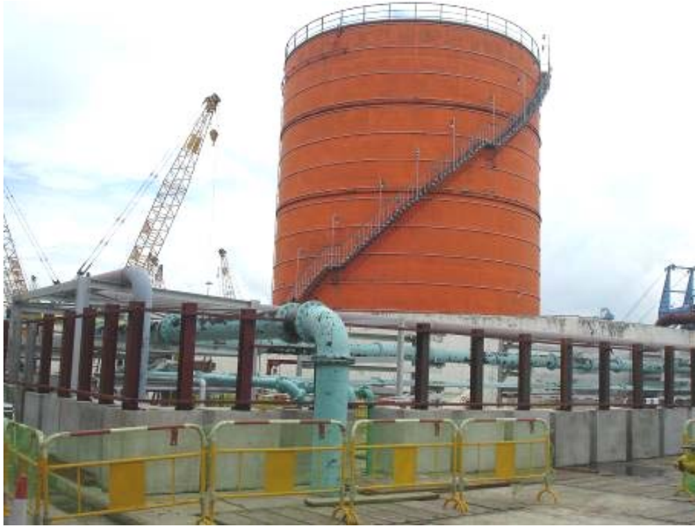
E. 3 Preparation works for demolition of existing Fuel Oil Day Tank
