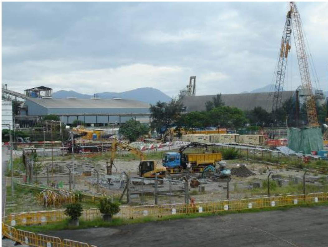
E.4 Demolition of existing Intermediate Pressure Reducing Station
