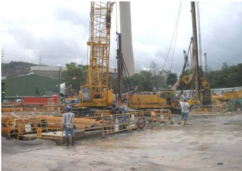
E. 2 H-pile works for Gypsum Handling Area
