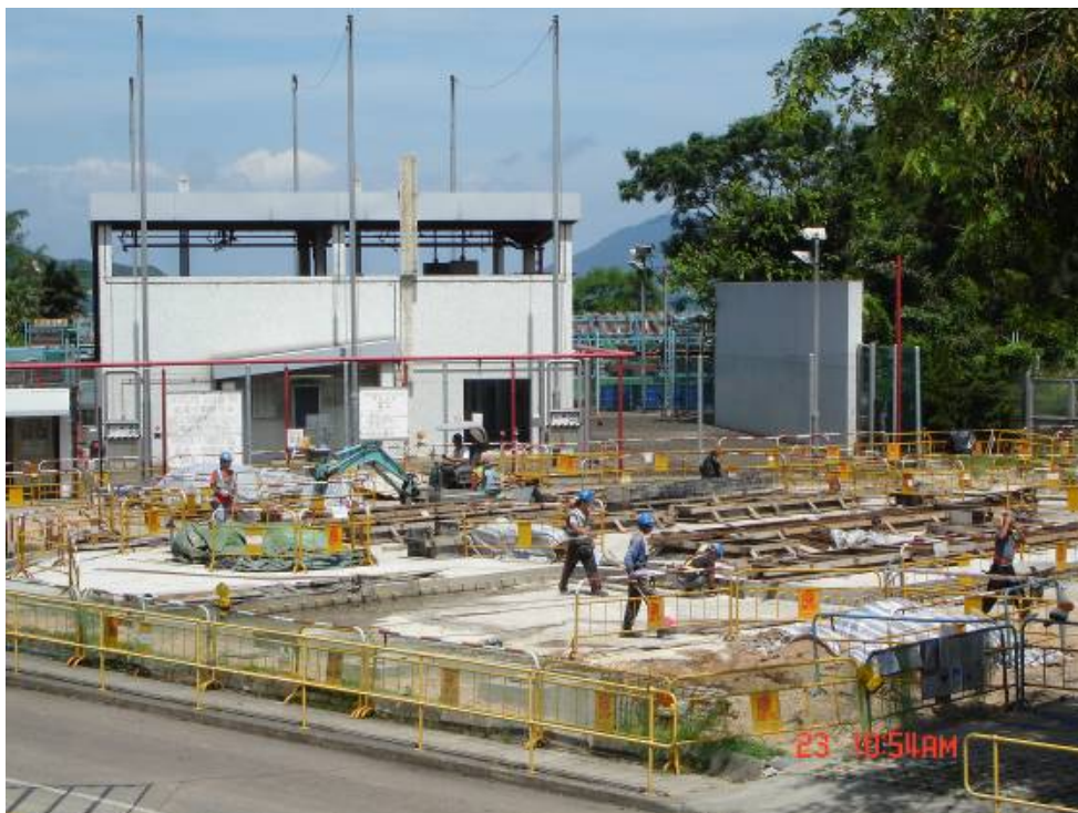
E.4 Foundation works for the new IPRS
