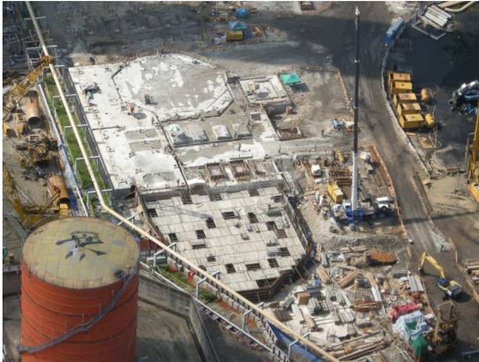
E. 1 FGD Absorber of Units B2 foundation work
