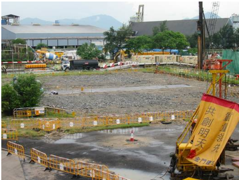
E. 2 Site clearance of ex-Intermediate Pressure Reducing Station (IPRS)
