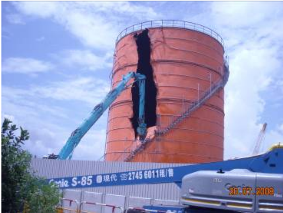
E. 3 Demolition of existing Fuel Oil Day Tank
