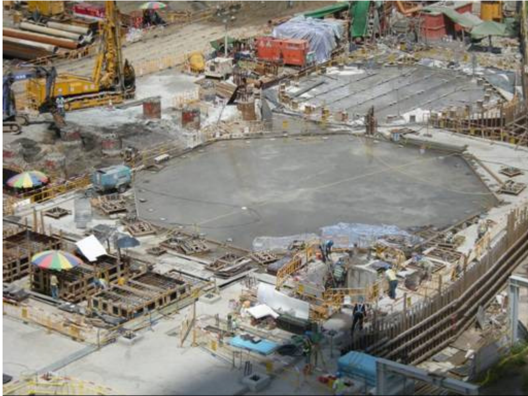
E. 1 Units B1 and B2 FGD Absorber foundation work
