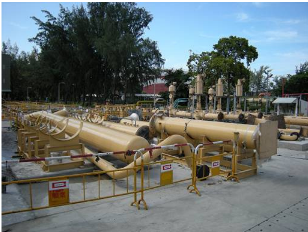
E. 2 Construction works for the relocated Intermediate Pressure Reducing Station
