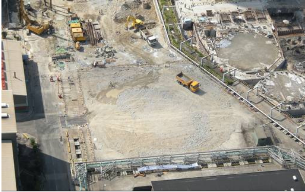
E. 3 Site clearance of ex-Fuel Oil Day Tank area
