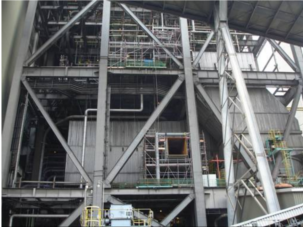
E.4 Mechanical erection works of Unit B1 NOx Reduction Facilities
