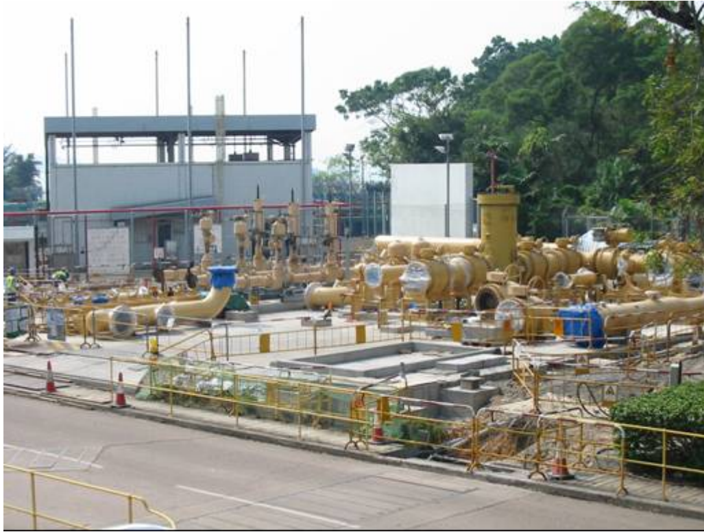
E. 3 Construction works for the relocated IPRS
