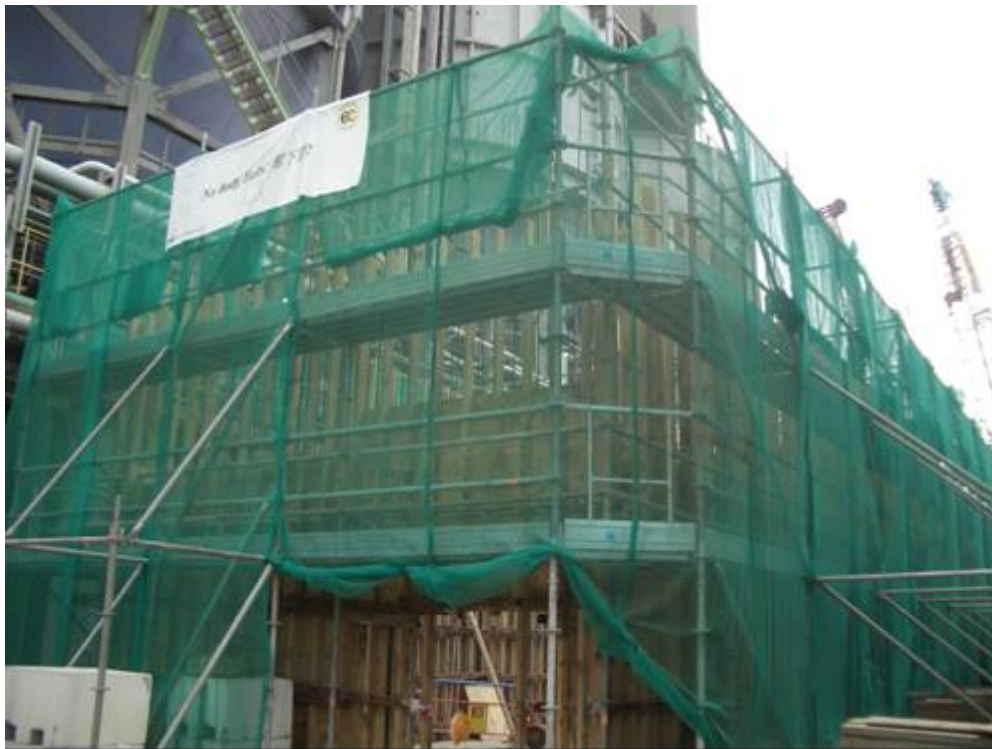
E. 2 EC Power Distribution Centre (PDC) construction
