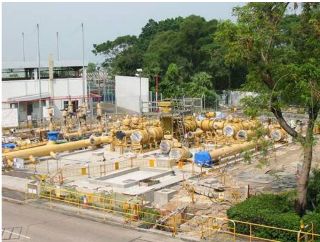
E. 4 Construction works for the relocated IPRS
