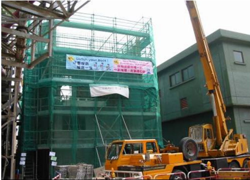
E. 3 EC Power Distribution Centre (PDC) construction
