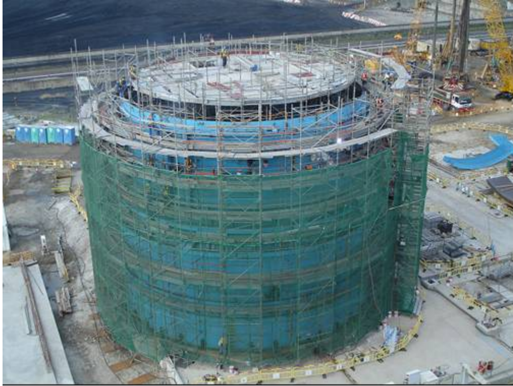
E.1 Mechanical erection works of Unit B2 FGD Absorber
