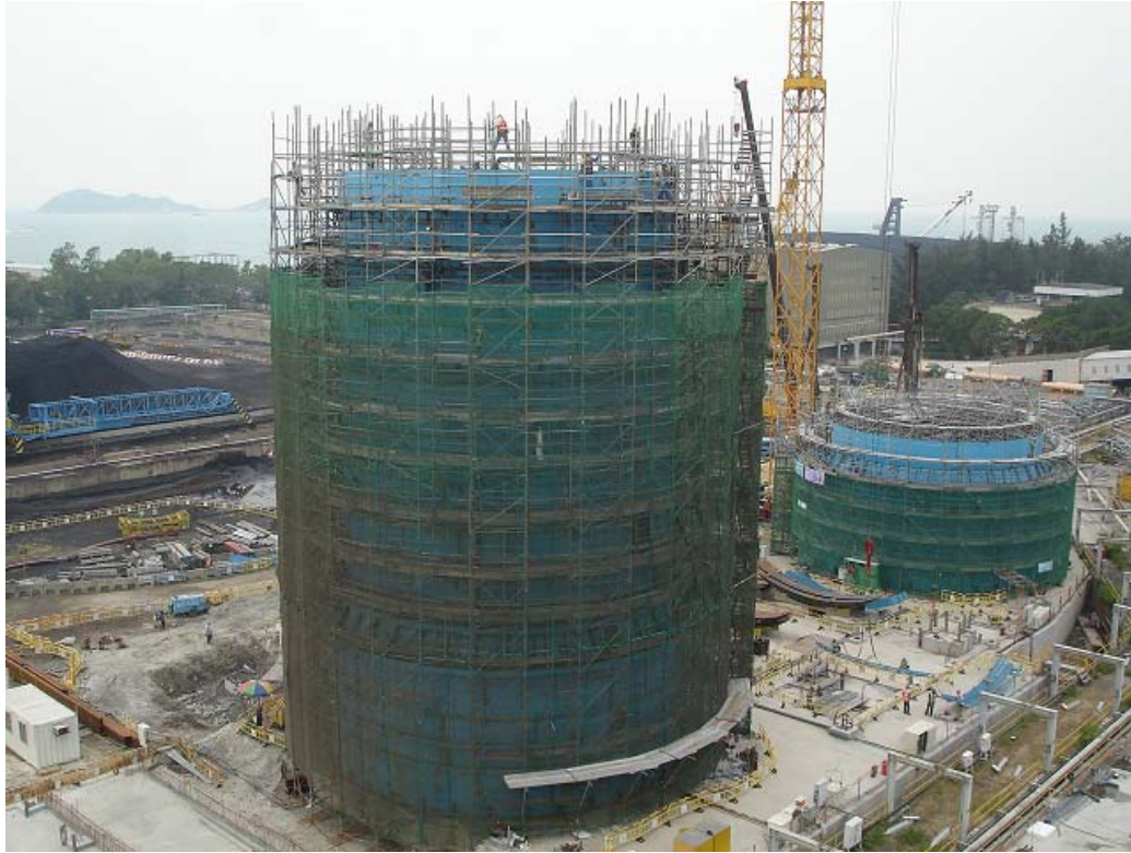
E.1 Mechanical erection works of Unit B1 and Unit B2 FGD Absorbers
