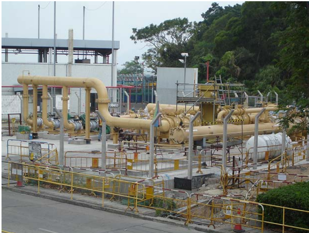
E. 4 Construction works for the relocated IPRS
