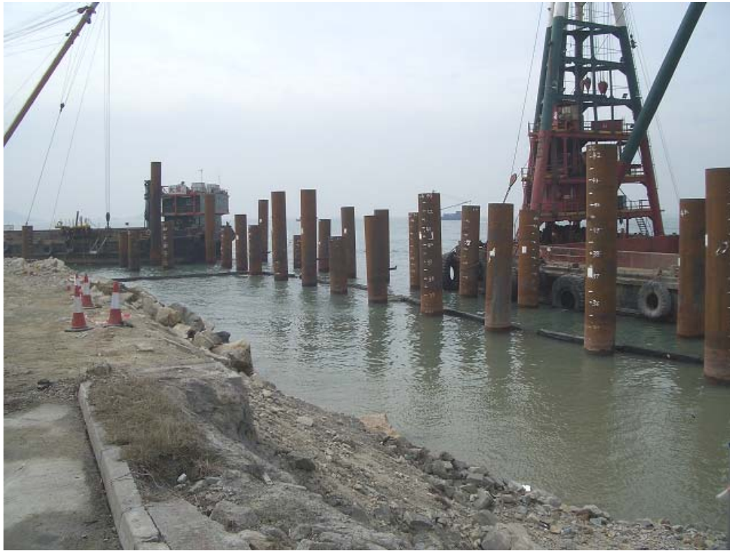
E. 3 Marine piling works for the Material Handling Berth
