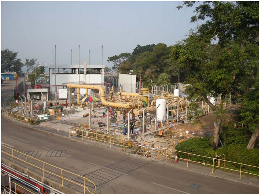
E. 4 Construction works for the relocated IPRS
