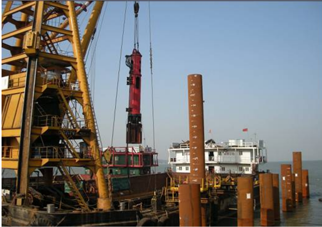
E. 3 Marine piling works for the Material Handling Berth
