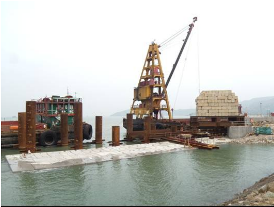
E. 3 Marine works at the Material Handling Berth
