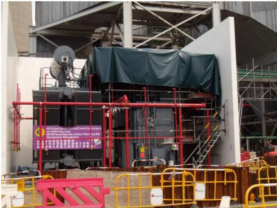
E. 4 EC Transformers installation works
