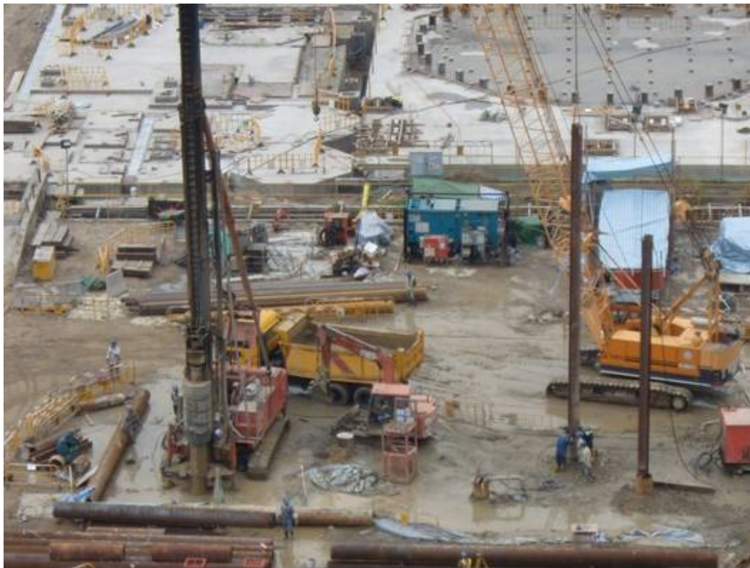
E.2 Piling works at Unit B3 and Unit B4 GGH area
