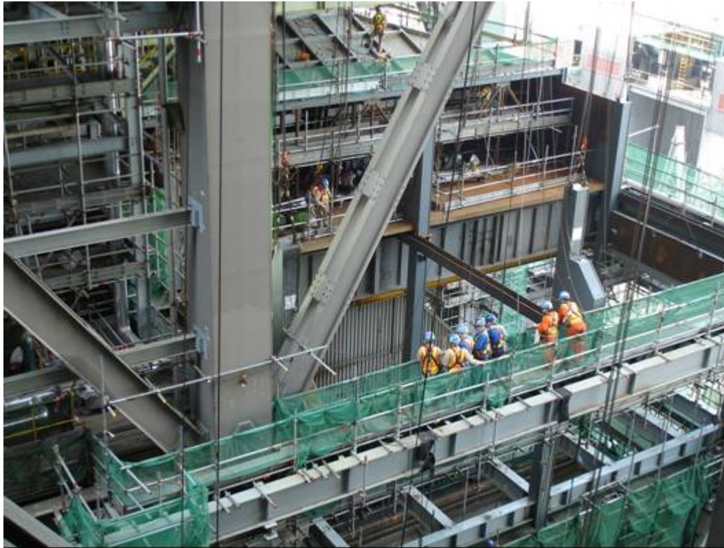
E. 3 Mechanical erection works of Unit B4 NO x Reduction Facilities
