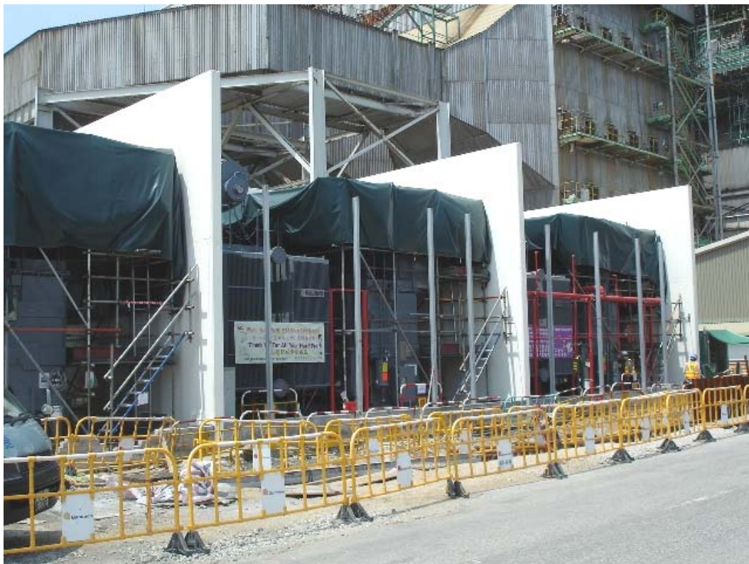
E. 4 EC Transformers installation works
