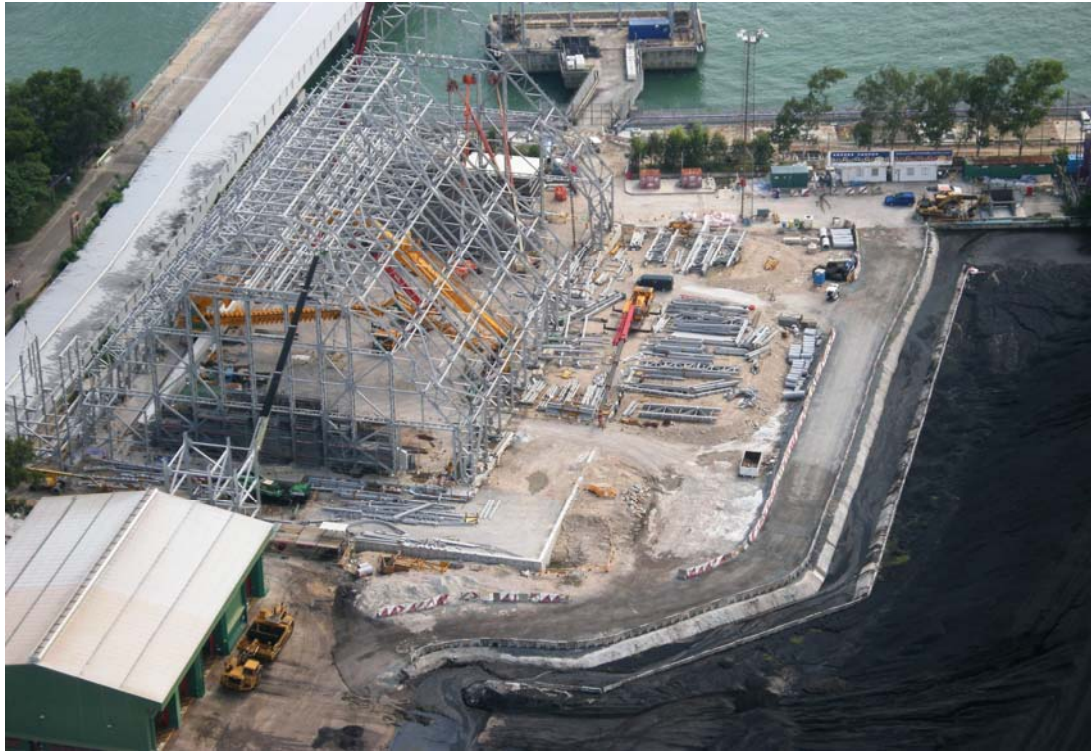
E.3 Gypsum Handling Area
