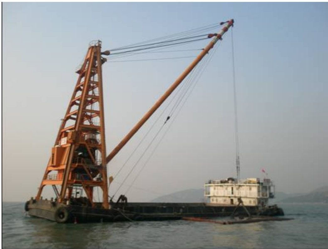
E.4 Dredging Work of Material Handling Berth
