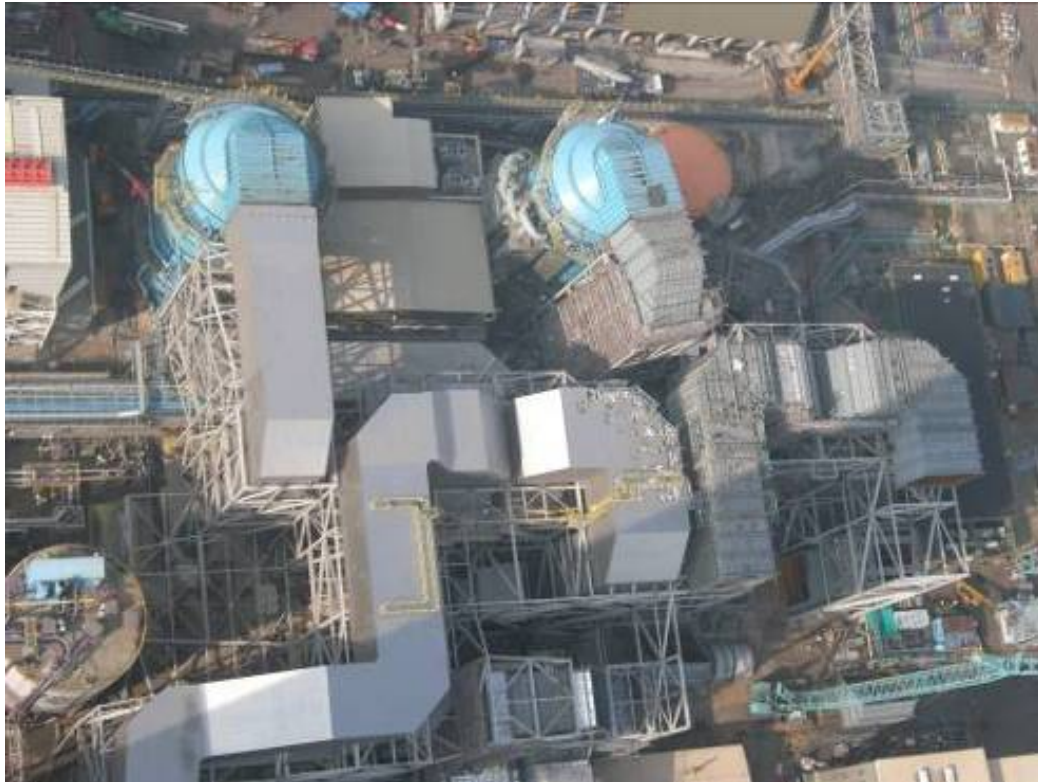
E.1 Unit B1 and Unit B2 FGD Areas
