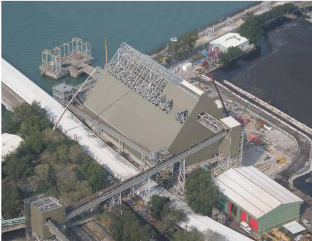
E.3 Gypsum Handling Area
