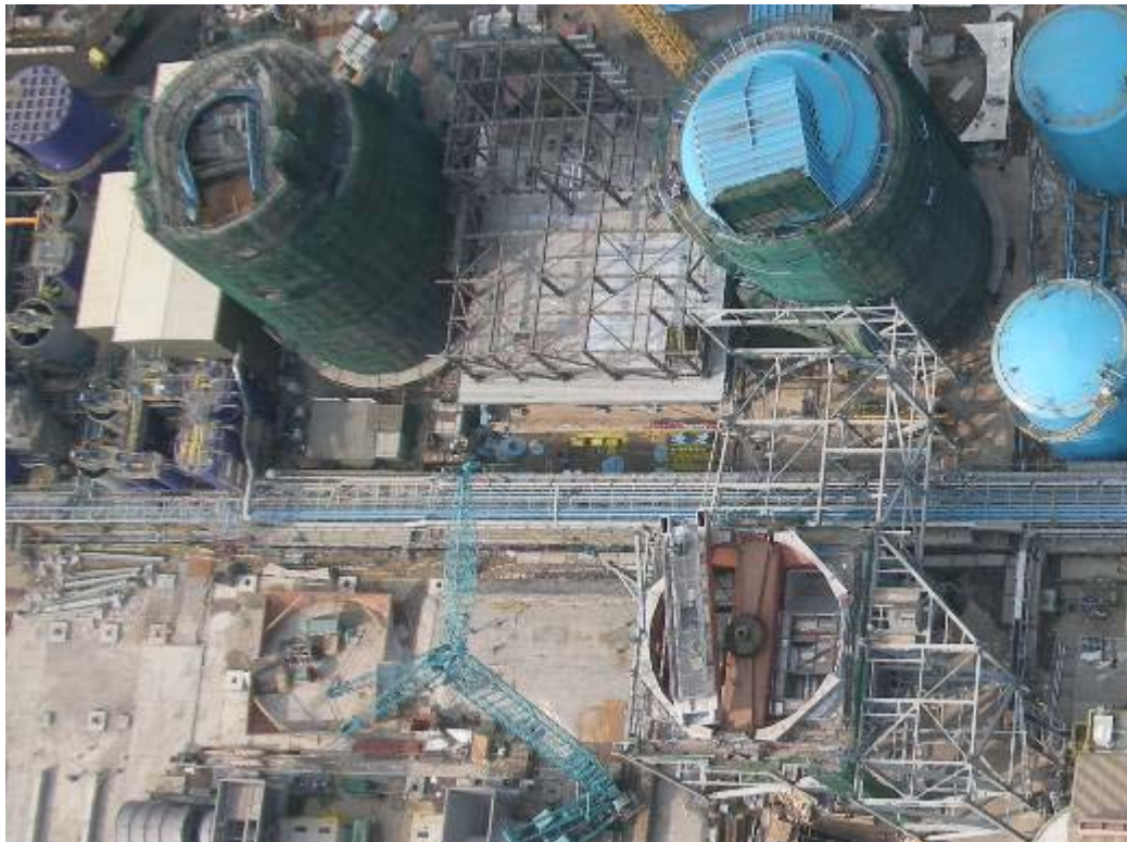
E.2 Unit B3 and Unit B4 FGD Areas
