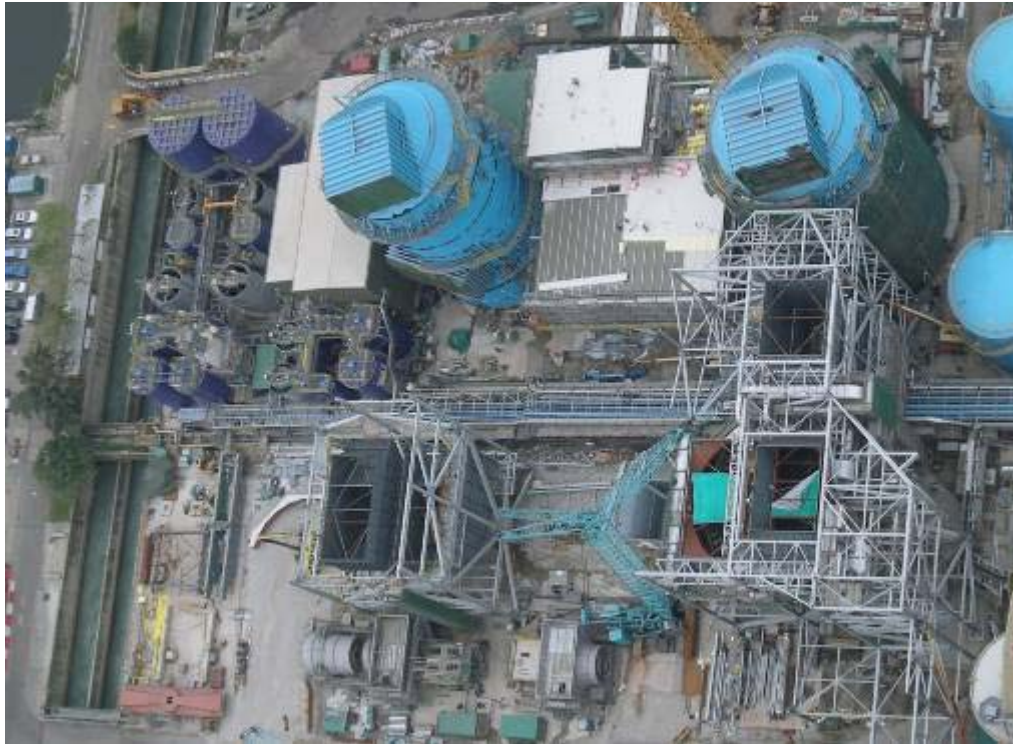
E.1 Unit B3 and Unit B4 FGD Areas
