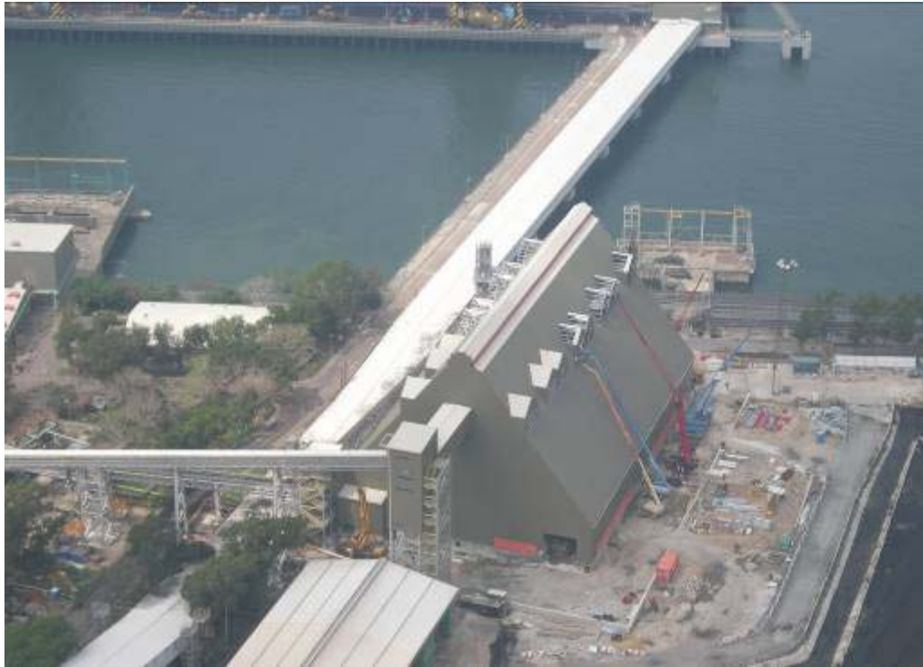
E.3 Gypsum Handling Area
