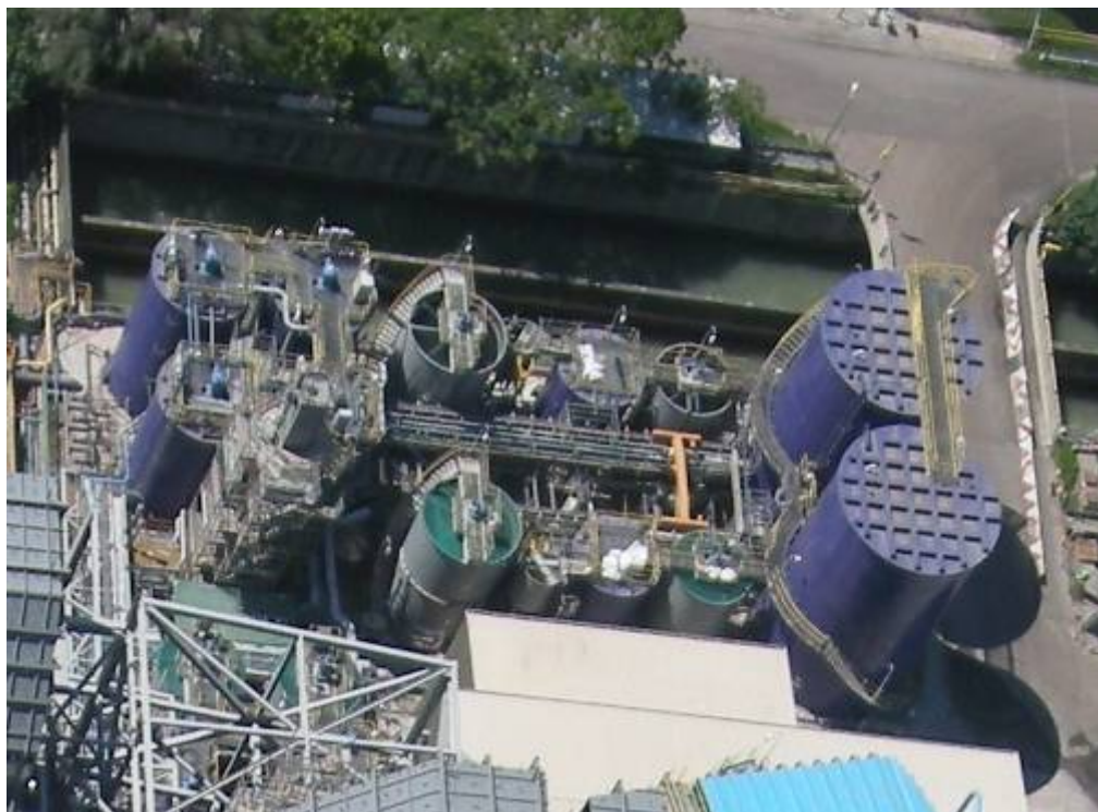
E.2 Waste Water Treatment Plant Area
