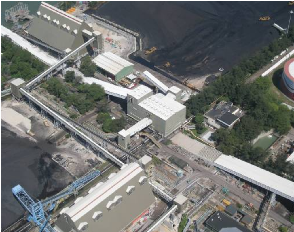
E.3 Limestone Handling Area and Gypsum Handling Area
