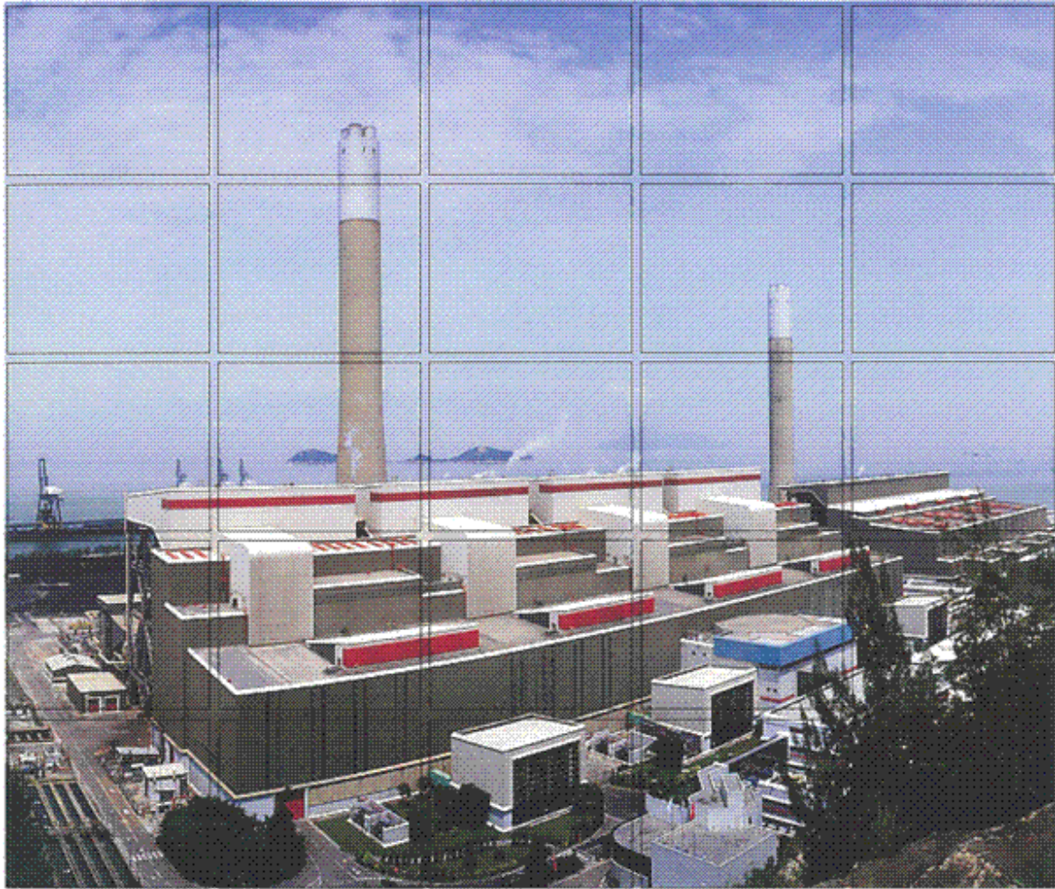
Emission Control Project at Castle Peak Power Station "B" Units
