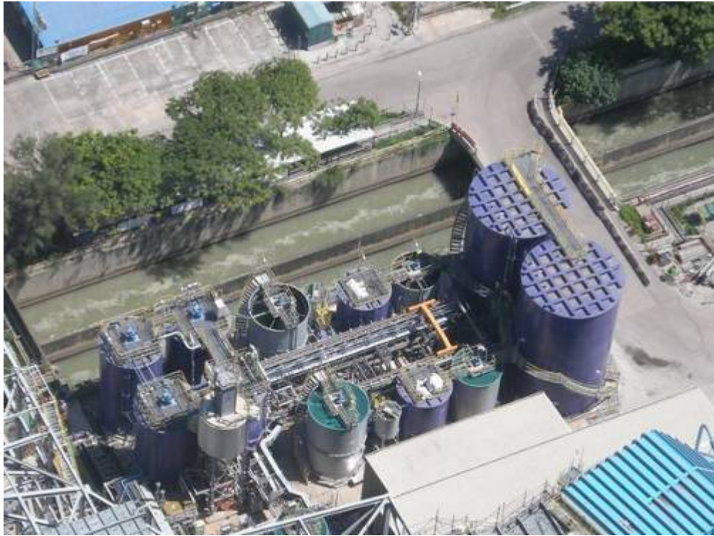
E.3 Waste Water Treatment Plant Area
