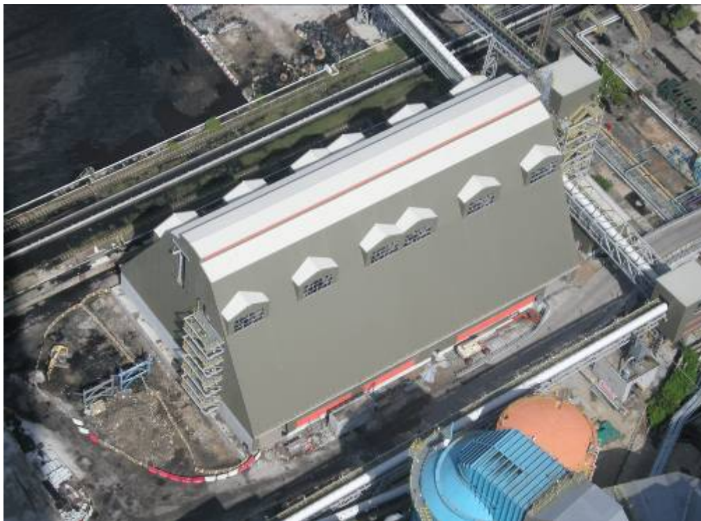
E.2 Limestone Handling Area
