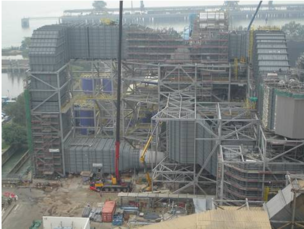
E.1 Unit B4 FGD Area
