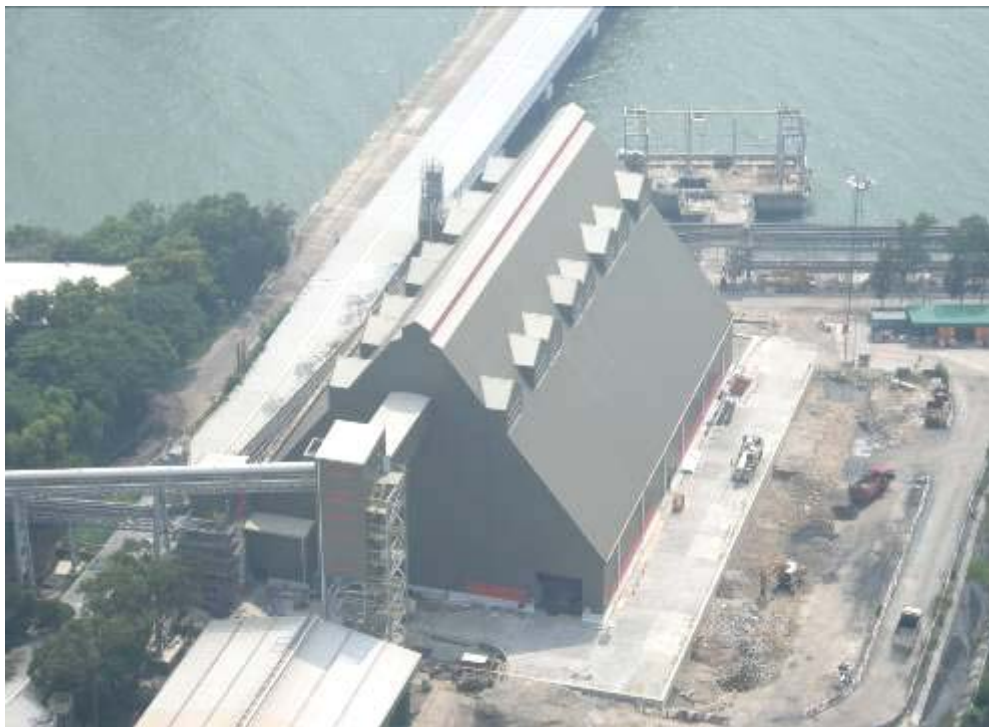
E.2 Gypsum Handling Area
