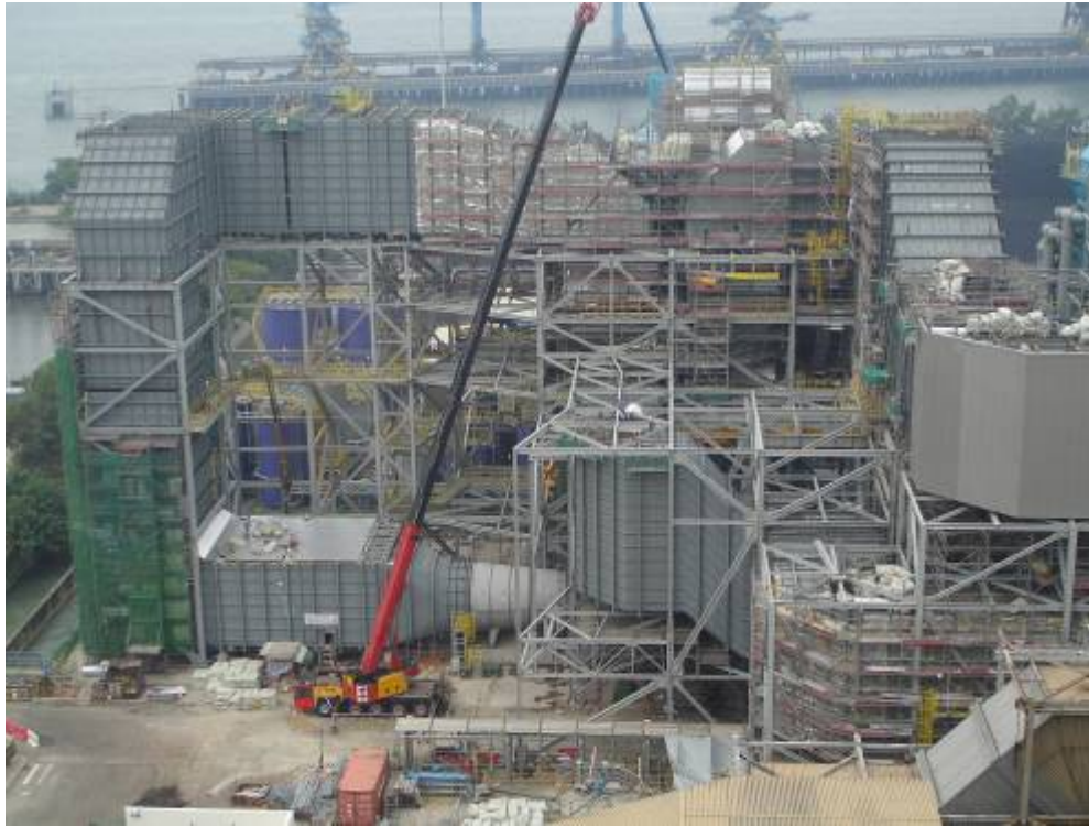
E.1 Unit B4 FGD Area
