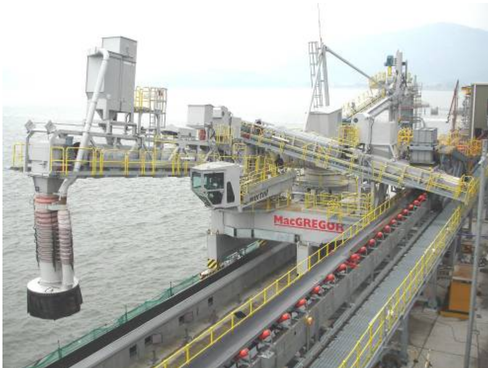
E.2 Loader/ Unloader at Material Handling Berth
