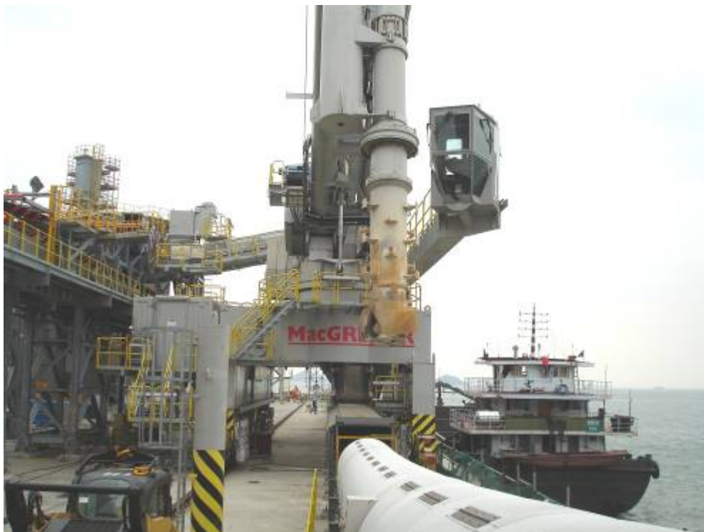
E.2 Loader/ Unloader at Material Handling Berth
