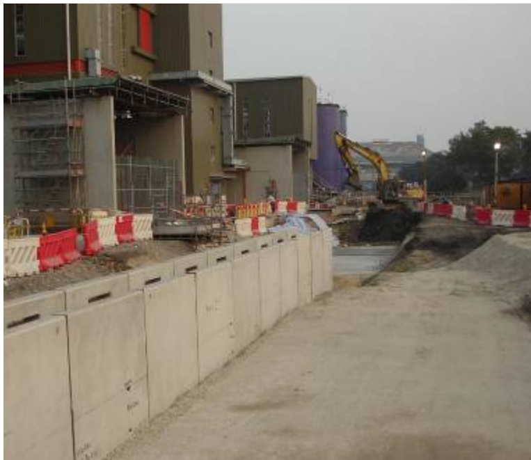
E.4 Civil Works
