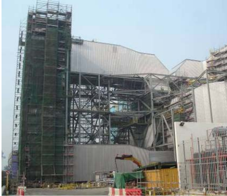
E.1 Unit B4 FGD Area
