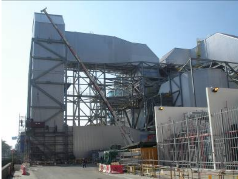
E.1 Unit B4 FGD Area
