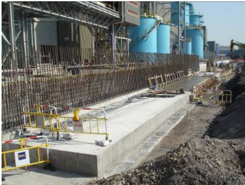
E.2 Civil Works
