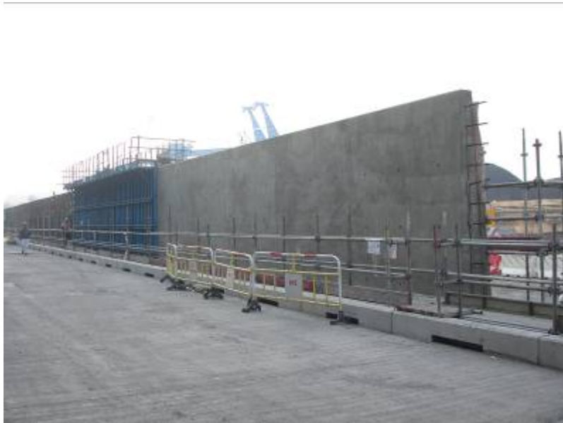
E.2 Civil Works
