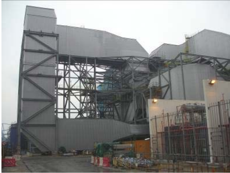
E.1 Unit B4 FGD Area
