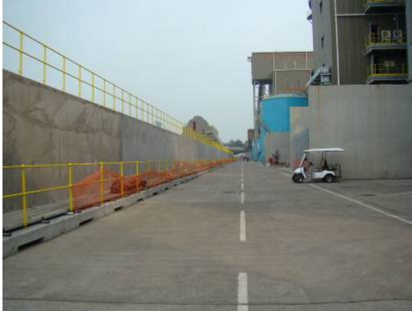
E.1 Completion of construction work for the retaining wall
