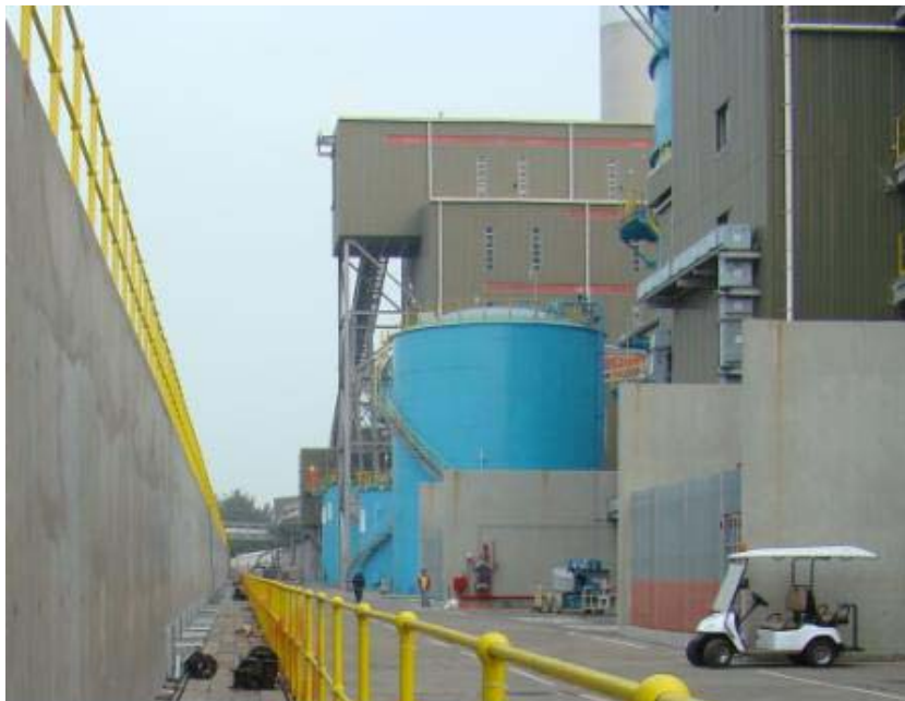
E.2 Building works at the retaining wall
