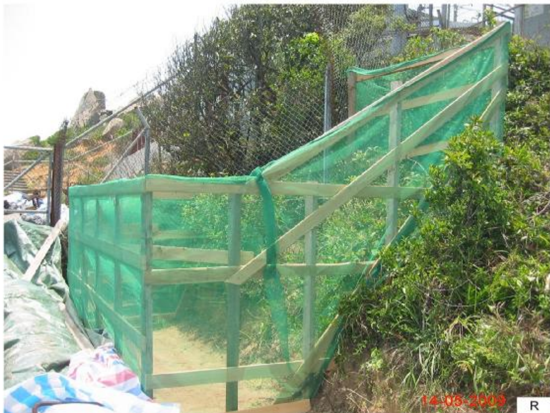
T2A and T3A Plant Protection Fence
