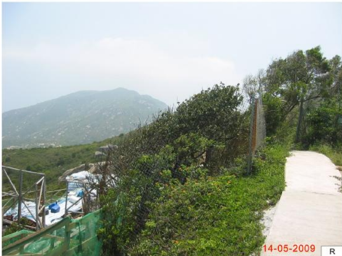
T1 with Tree Protection Fence
