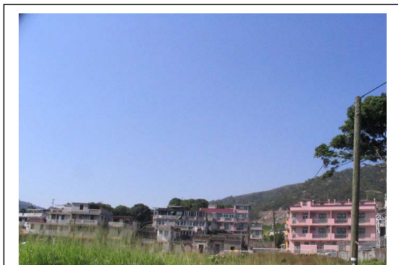
Photo No. C10—R3
