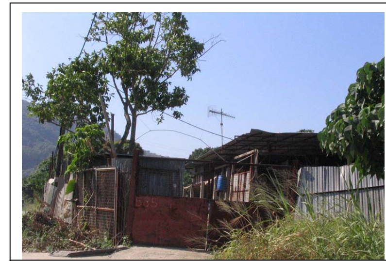
Photo No. B12—LCA 6 Industrial Landscape Character Area
