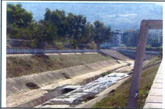
Photo No. B13—LCA 7 Nallah Landscape Character Area
