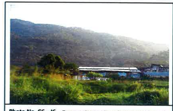
Photo No. C6-16 Temporary Structure for poultry and Open Storage at upstream of Ma On Kong Channel
